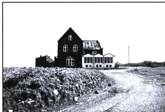
The Haven Fort Hotel, with the circle where the object was seen still visible.
